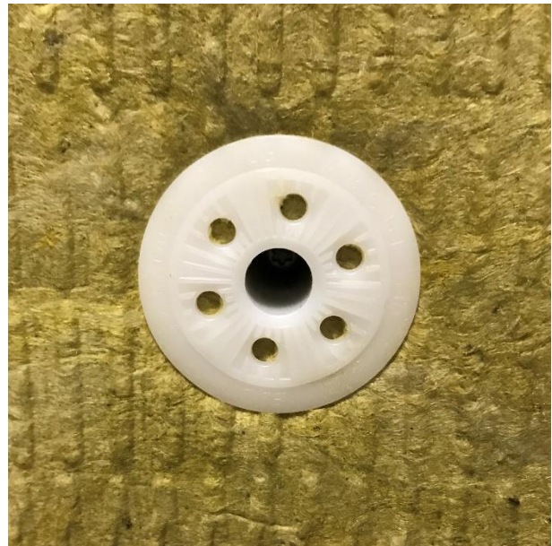
Fastener screw tightened with washer slightly indenting in to the surface of the insulation
