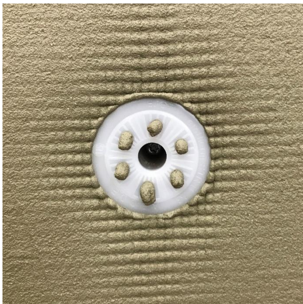
Fastener screw tightened and washer head sitting flush with the base coat surface
