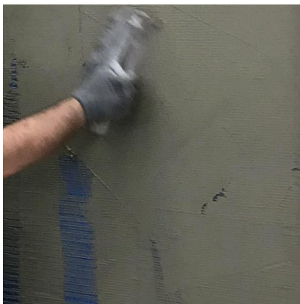
Reinforcing mesh embedded into the surface of the first layer of base coat
