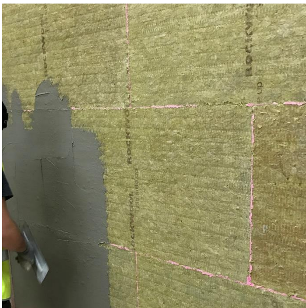
A tight skim coat of base coat applied to the surface of all the insulation boards
