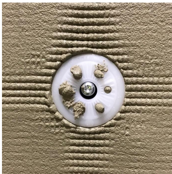
Fastener lightly tapped into the render surface
