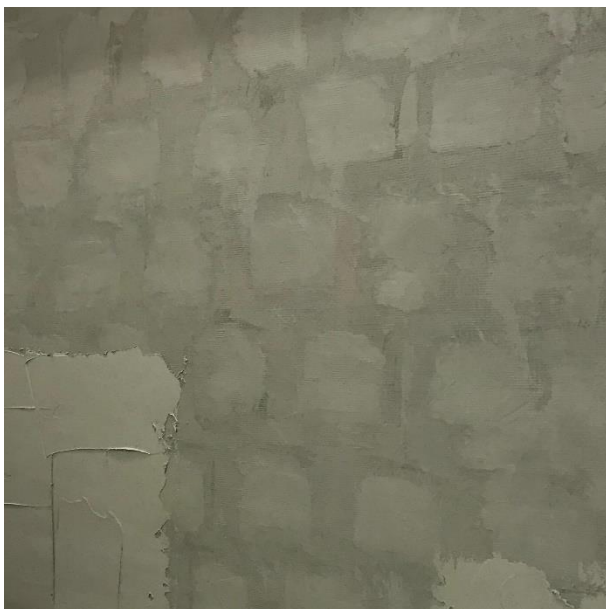
Second pass of base coat applied over fasteners and mesh patches
