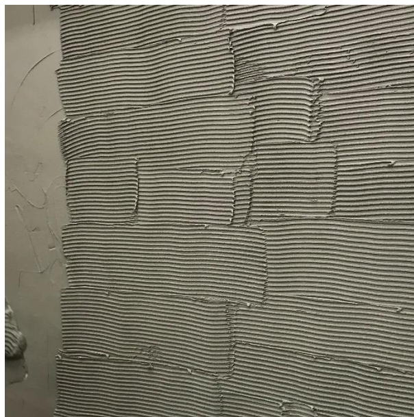
Second coat applied with a notched trowel at a nominal 3 mm to achieve a total overall 5 to 6 mm base coat thickness
