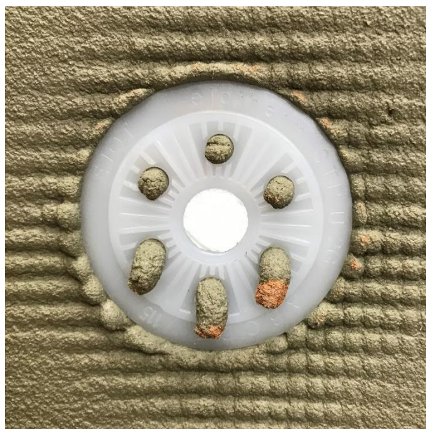
Plug used to fill the recess in the head of each fixing
