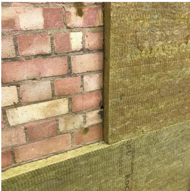
Insulation board pushed back to the substrate with a minimum 200 mm overlap between board joints
