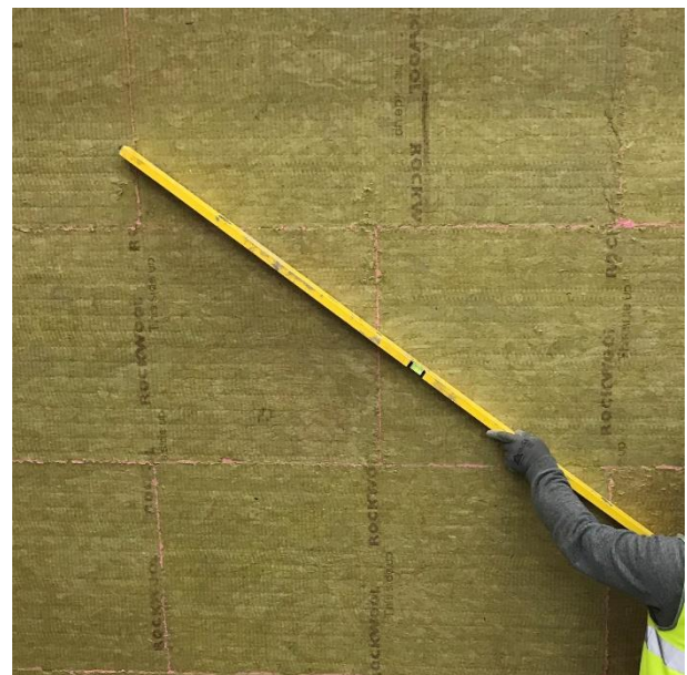
Flatness of the installed boards checked using a level or straight edge
