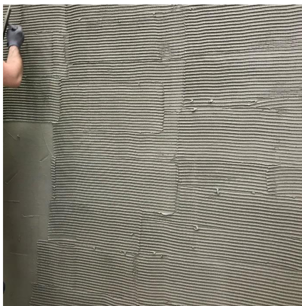
First pass of base coat applied with an 8 mm notched trowel to achieve a nominal 3 mm first coat
