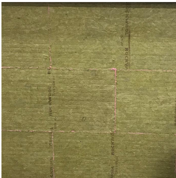
Overview of board installation with filled board joints
