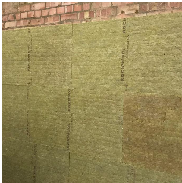
Boards installed in a brick bond pattern
