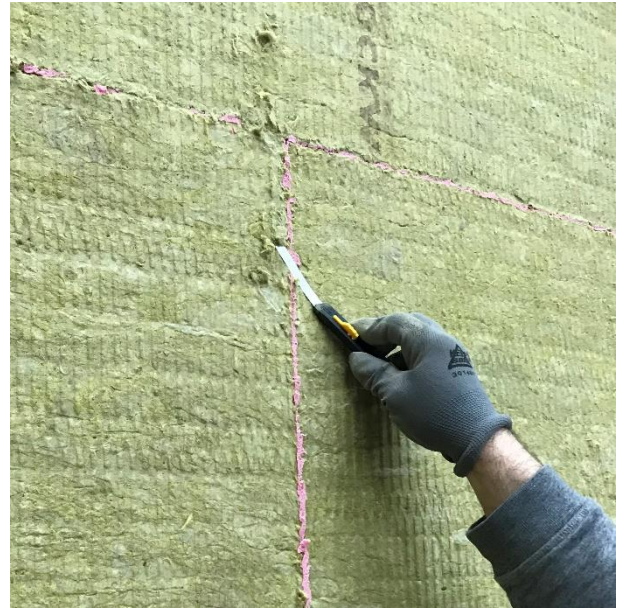
Foam left to cure and cut flush with the board surface
