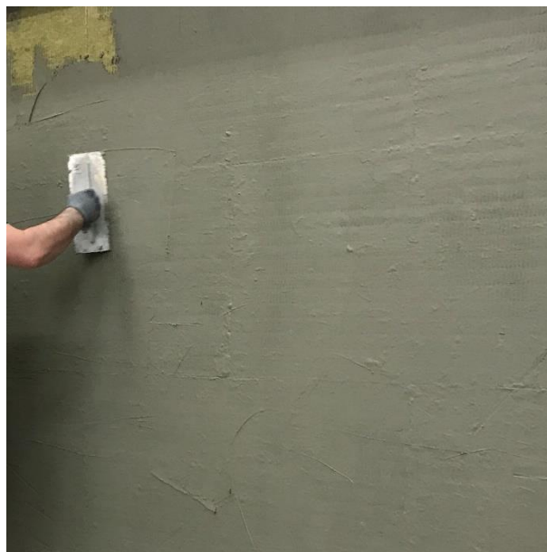
Skim coat applied ready to receive first pass
