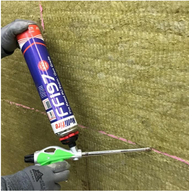
Board joints filled with expansive foam
