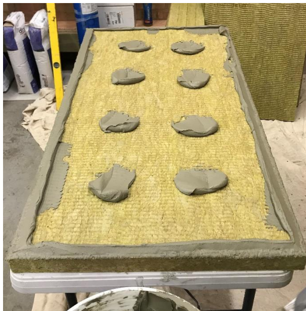
Ribbon and dab application of adhesive to the back of the insulation board
