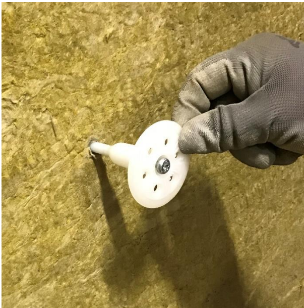
Hole drilled through the board in to the substrate with a masonry drill of the correct size and embedment depth
