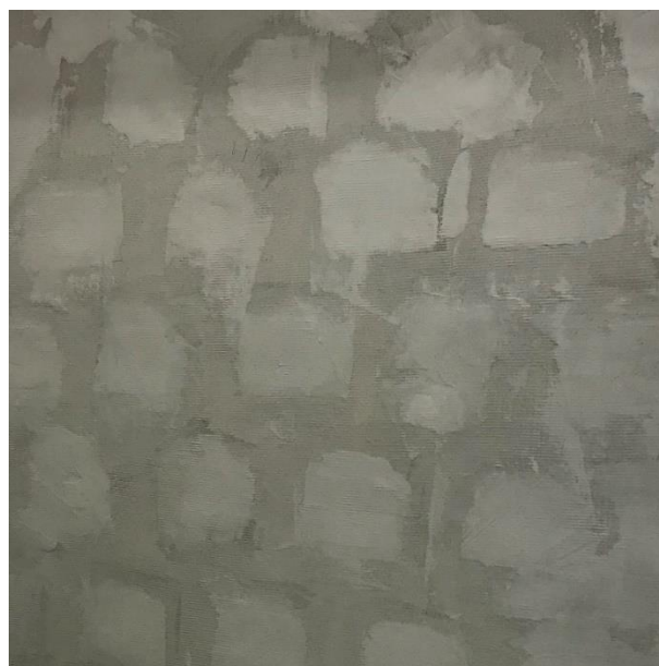
All mesh patches fully embedded in base coat
